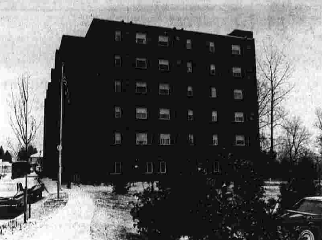
Raymond L. Miller Gardens, a six-story highrise with 84 one-bedroom apartments for elderly single people, stands about half a block east of Main St. opposite the Coca-Cola Bottling Co. in East Hartford. Town officials and leaders of the Housing Authority dedicated the building Saturday afternoon.
